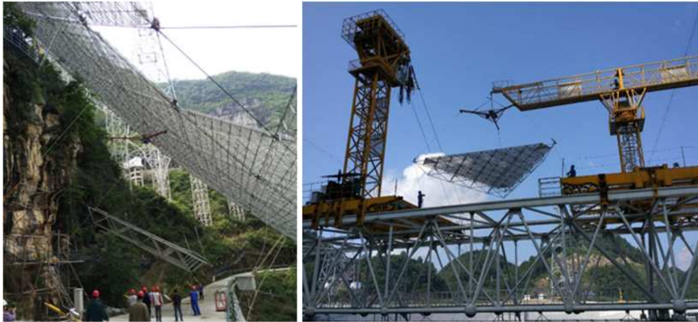
Fig. 13 Photos of maintenance scheme for reflector.
