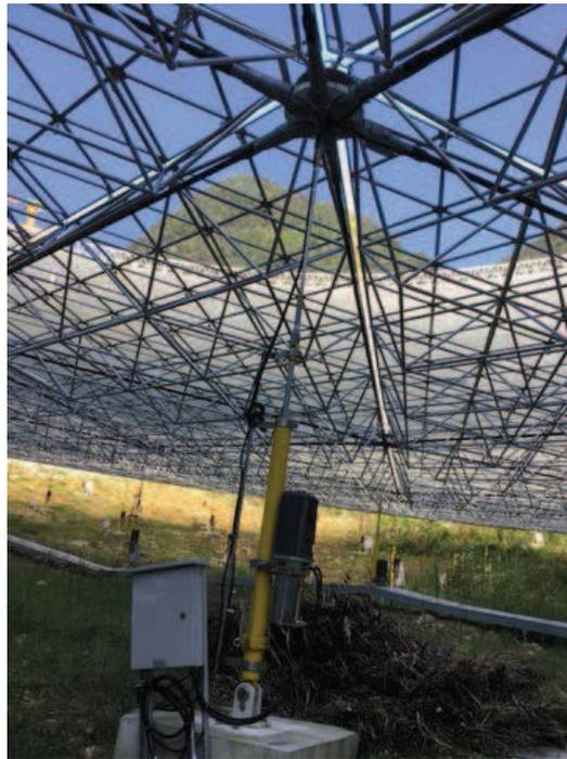
Fig. 2: One actuator connected to its node plate.
